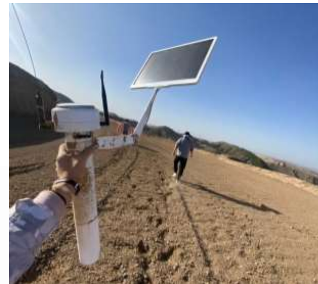
Fig. Install rain gauges at the CW
